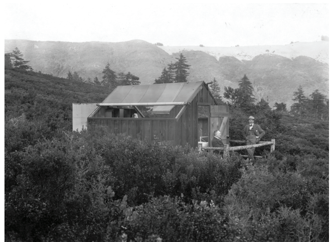
Circa 1912 canvas-roofed cabin at Muir Woods, built near the Sierra Trail. Guests could roll up the roof and see the night sky. Note cast iron bed frame in cabin doorway and the view through open roof to cabin beyond. Canvas shower enclosure visible at left.
